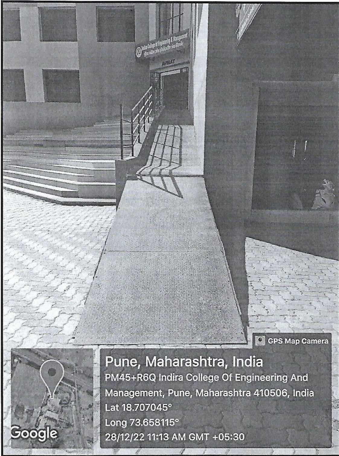
Photo 03: Ramp at Avirat Entrance
