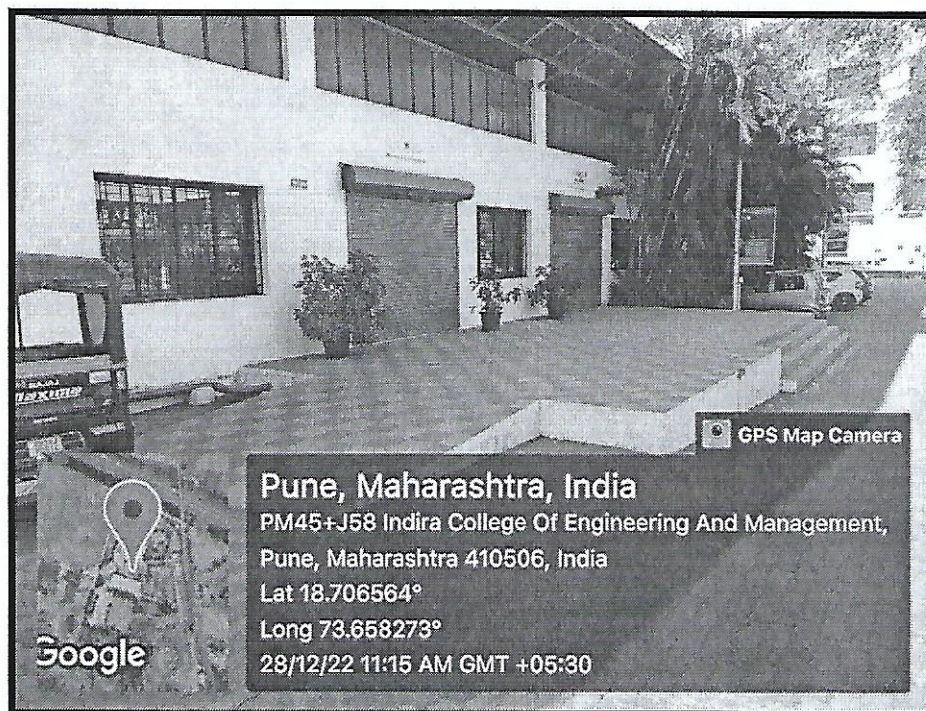
Photo 02: Ramp at Workshop Entrance
