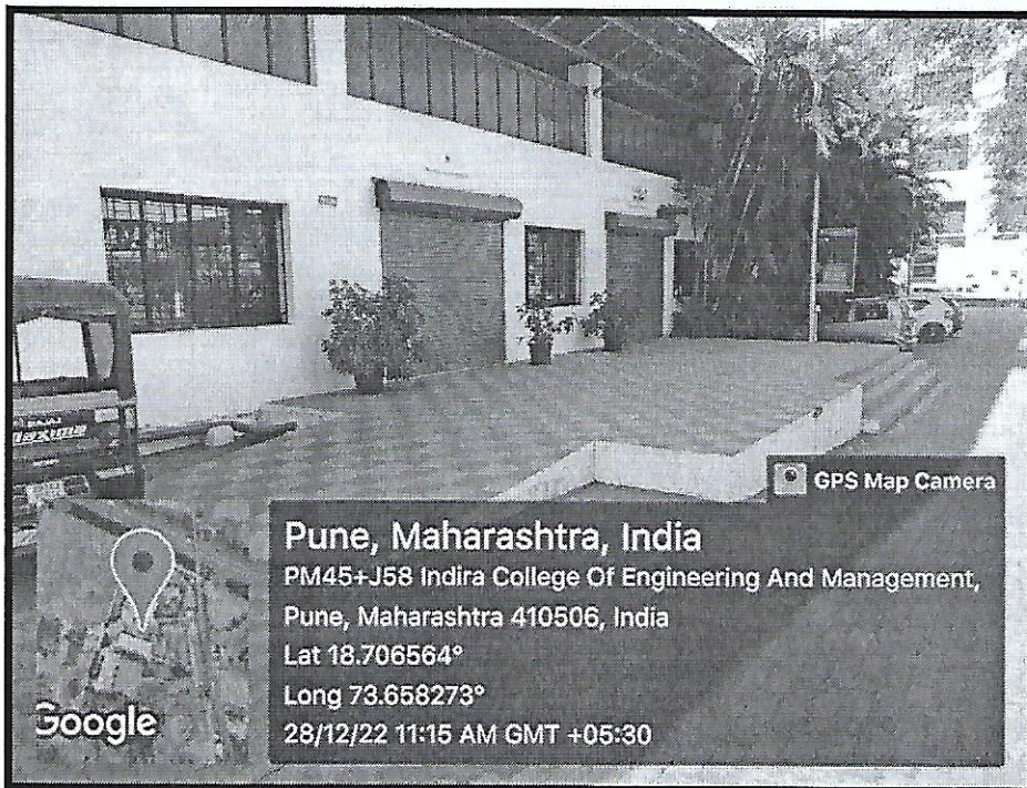
Photo 02: Ramp at Workshop Entrance
