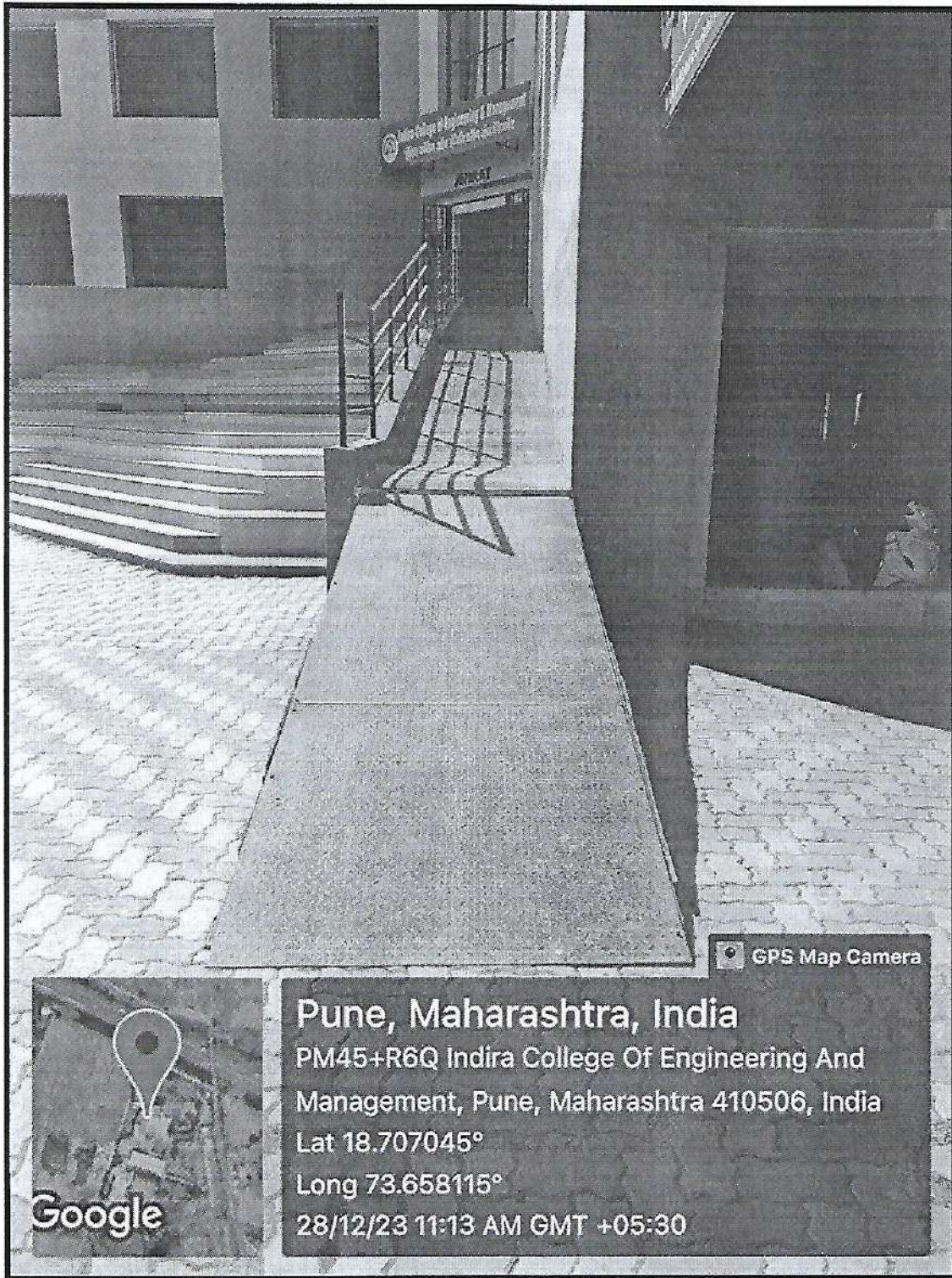
Photo 03: Ramp at Avirat Entrance
