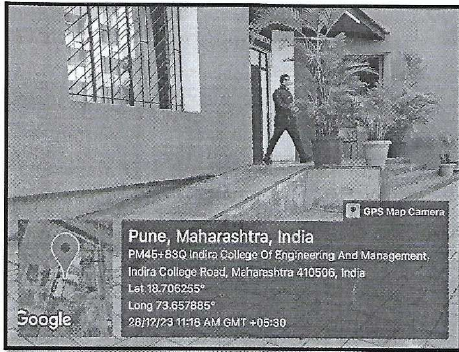
Photo 01: Ramp at Admin Building Entrance
